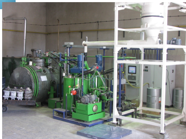
Vacuum Casting : Part of Medium Voltage Production Line
